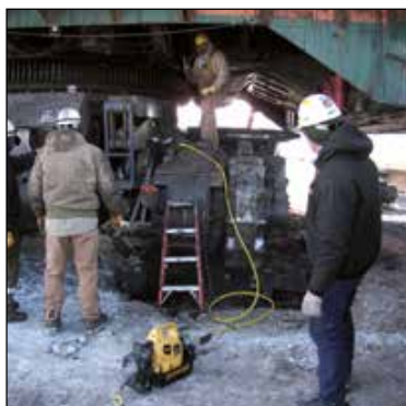
◀ Any brand of hydraulic torque wrench can be powered by the portable ZU4-Series torque wrench pump.
